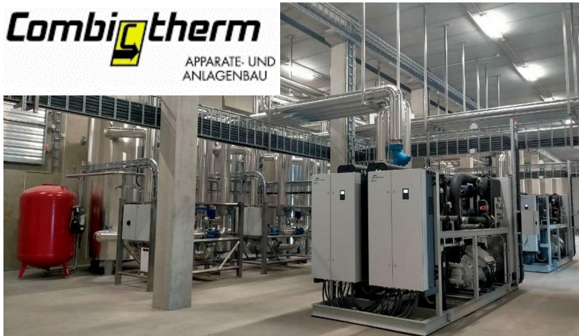
4 x HTHPs from Combitherm (3.5 MW heating capacity, R1233zd(E), screw compressor from Bitzer) use the dryer exhaust air as a heat source and generate 120 °C via an intermediate circuit to heat the drying air
